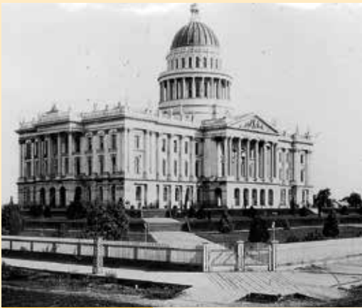
State Capitol, CA. 1875 - today, tens of thousands of visitors to the State Capitol are able to see how state government offices looked in the early 1900's.
